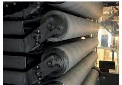
Tower filter belts
